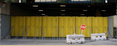
LOADING DOCK DEPLOYABLE FLOOD GATE
