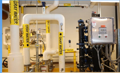
SCIENCE BUILDING GREY WATER RECYCLING SYSTEM
