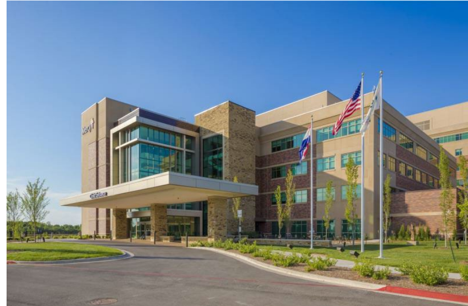
Mercy Hospital Joplin, which opened in March 2015. The new hospital is a "storm-hardened" facility with a precast concrete shell, windows that can withstand high winds, and partially buried generators for backup power in an emergency.
