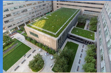
12,000 SF GREEN ROOF
